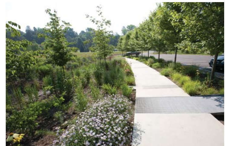
Bioswales, similar to drainage ditches, utilize selected vegetation to filter and slow down stormwater runoff prior to its drainage into the water shed. These bioswales can be designed using native vegetation adapted to the area, requiring minimal maintenance.
