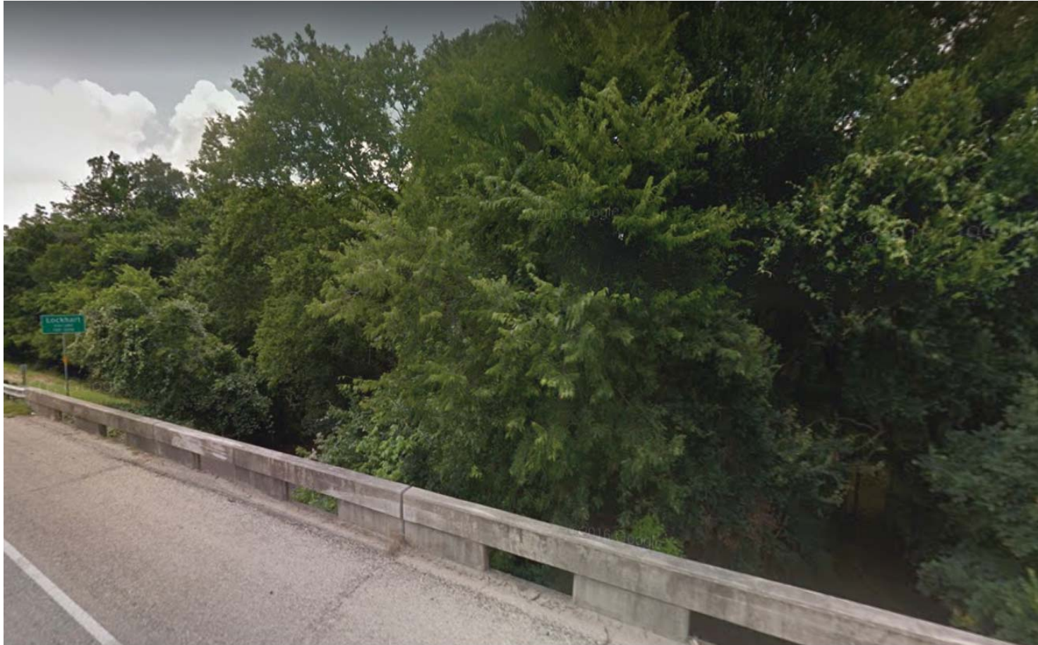
View of Comanche Ridge Park property frontage from the bridge over Plum Creek.
