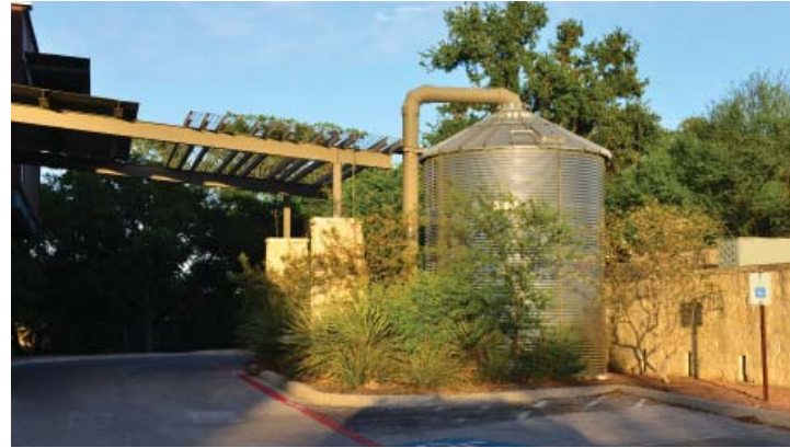
Rainwater harvesting should be considered during the development of future pavilions. The above example captures rainwater from a pavilion roof top and stores it in a 5,000 tank for use in irrigation of the park landscape.
