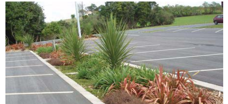
Use of native plants within landscape areas of parking lots can aid in removal of contaminants and sediments from stormwater prior to drainage into the watershed.
