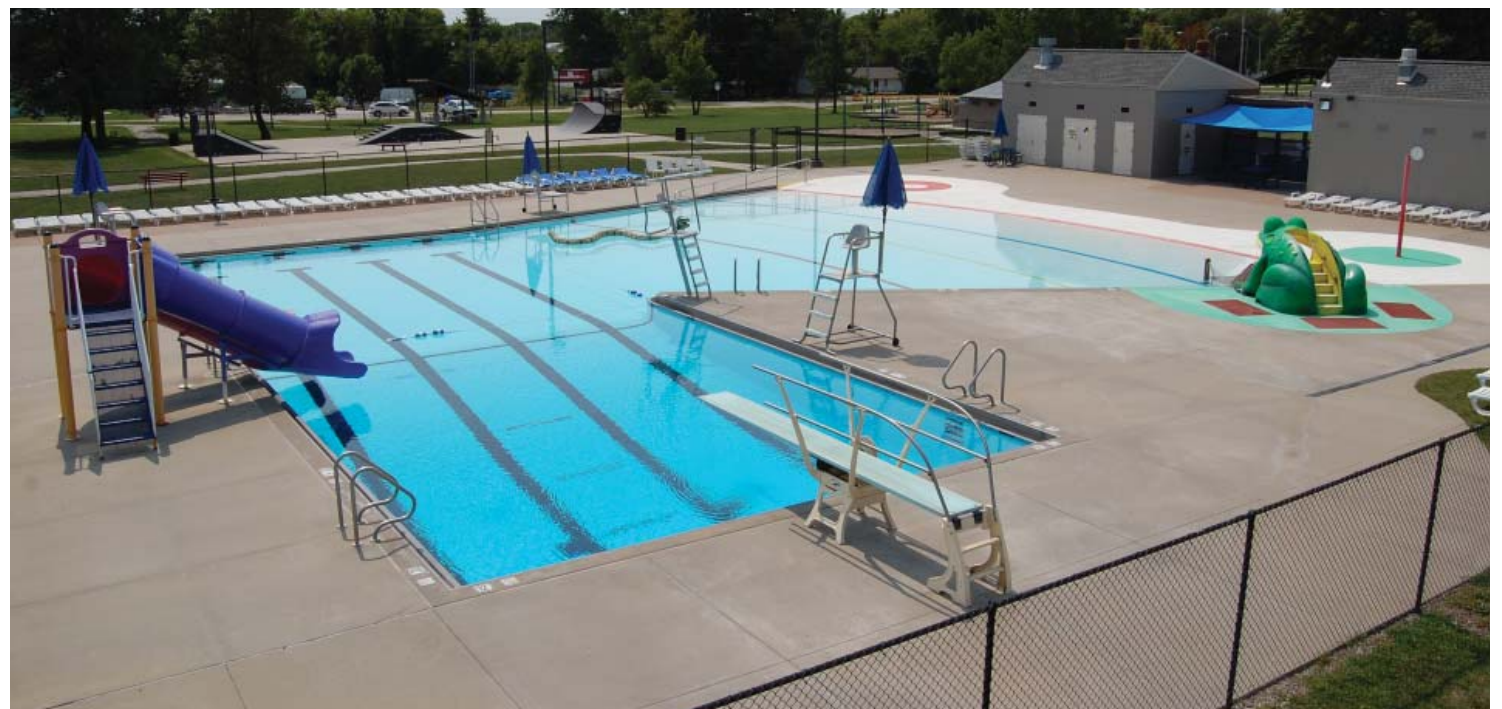
Modern zero-depth entry pools cater to a wide range of users, providing ease of access to the water for young children and senior citizens or users who may be more comfortable in shallow-water environments. Existing pools can be renovated to include this style of shallow area while retaining traditional competition/lap lanes. (source: City of Grain Valley, MO)
