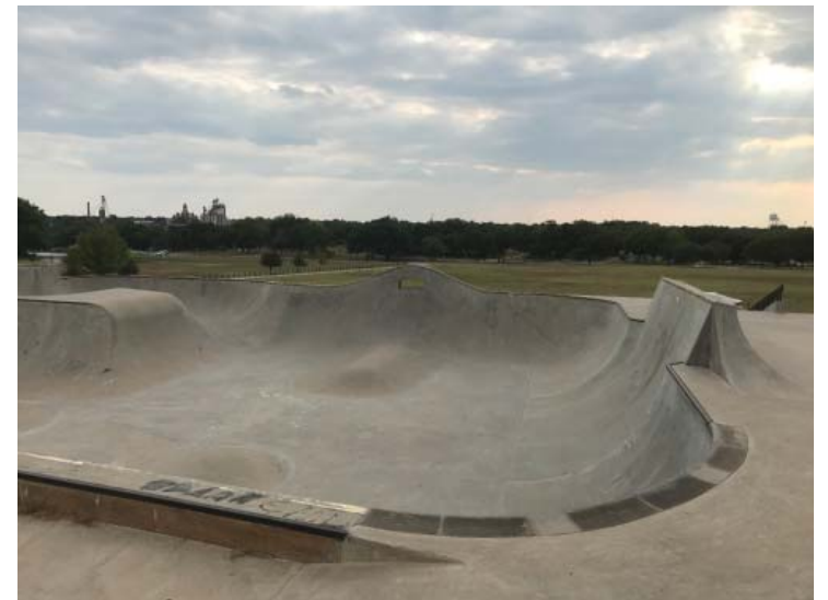
The Lockhart Skatepark is a poured-in-place concrete facility that offers a variety of vertical and street elements for skaters of all ages.
